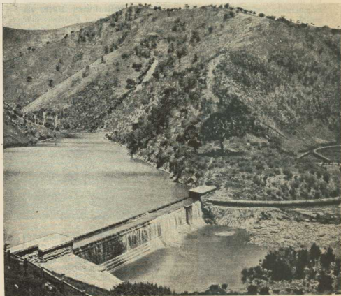
Abb. 4. Staudamm in Queensland.
